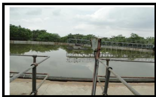
Figure 14-20: secondary clarifier
