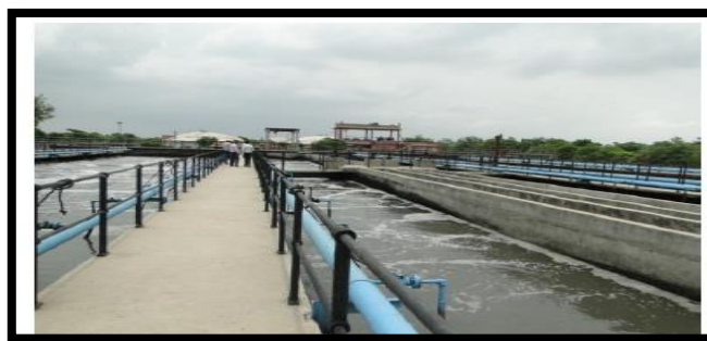
Figure 14-19: Aeration tank
