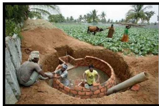
Figure 8-2: Construction of Bio Gas Plant
